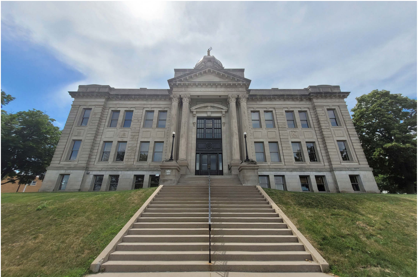
In 2020 and 2021, Jackson County's historic courthouse was refurbished with $2.5 million in wind revenue funds. This project included fixing and replacing the copper dome and statue on top of the building, roof work, and tuck pointing.
