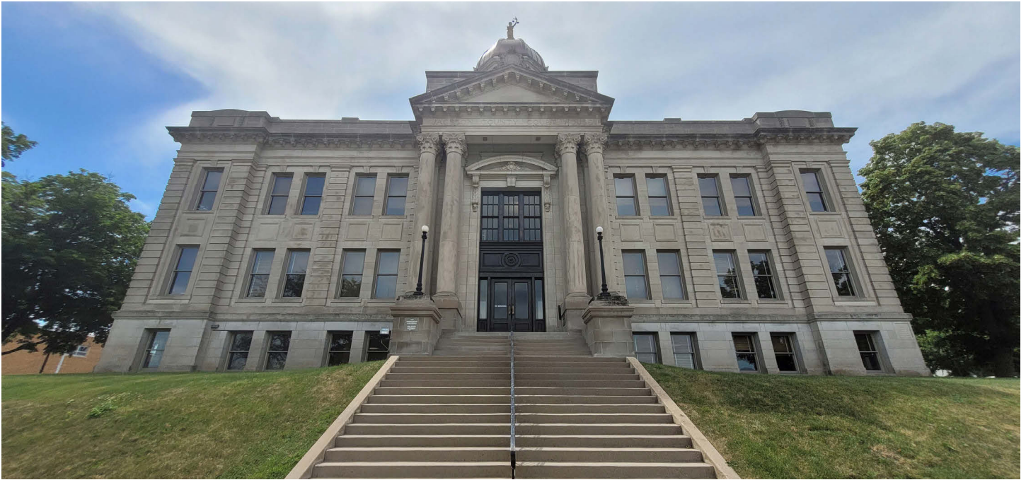
In 2020 and 2021, the historic courthouse in Jackson County, Minnesota, was refurbished with $2.5 million in wind revenue funds. This project included fixing and replacing the copper dome and statue on top of the building, roof work, and tuck pointing. | Photo by Molly Malone
