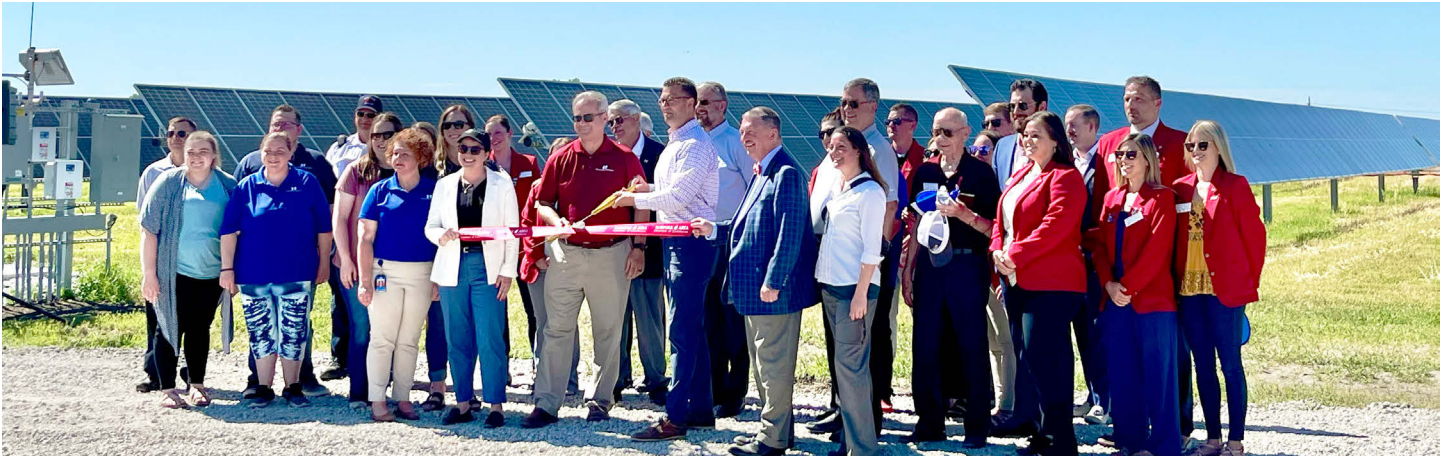
Early this summer, officials celebrated the opening of a community solar development in Norfolk, Nebraska. The project is the largest in the state at 8.5 megawatts on 75 acres. | Photos by Lindsay Mouw
