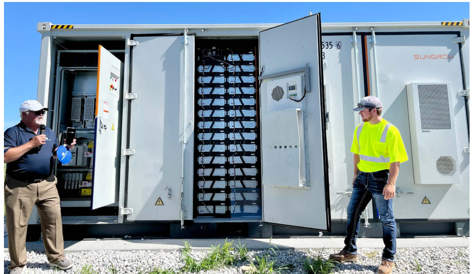
The community solar site in Norfolk, Nebraska, features a 1.5 megawatt energy storage battery that discharges power during peak energy demand.
