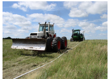
Figure 10: Pipeline installation in Thedford, Neb. | Photo by Don Earl
